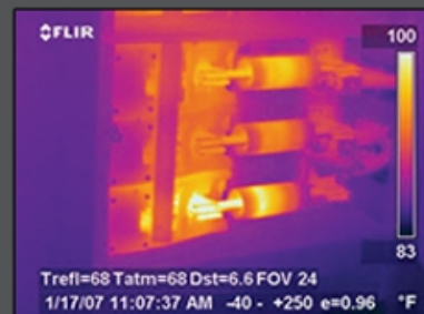
Figure 1 - Hot Fuse Connection
